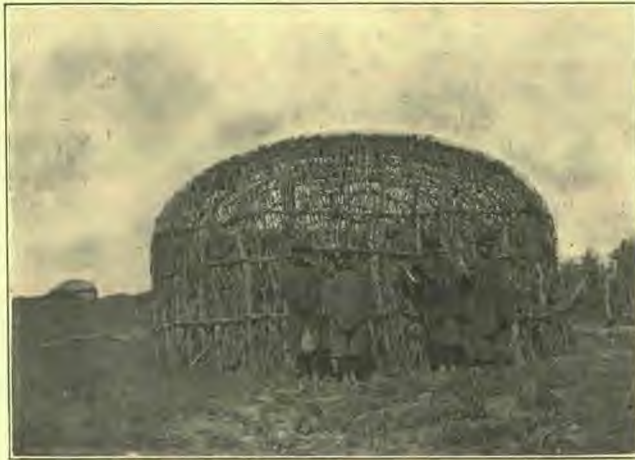
THE FRAME-WORK OF A KAFIR HUT.
