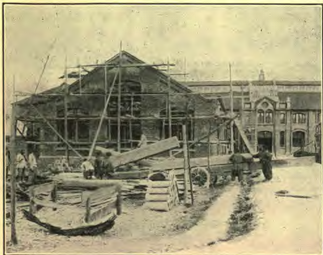
"Our new photoengraving building. The large timbers are being brought in to be sawed into lumber by hand, as there are no sawmills here"
