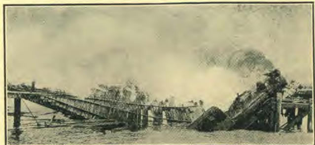
WRECK CAUSED BY THE BREAKING OF WORM-EATEN PILES
