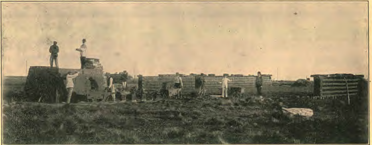
MAKING BRICK FOR THE NEW DORMITORY TO BE CONSTRUCTED WITH THE MEANS RAISED BY THE SABBATH-SCHOOLS ON DEC. 28, 1912
