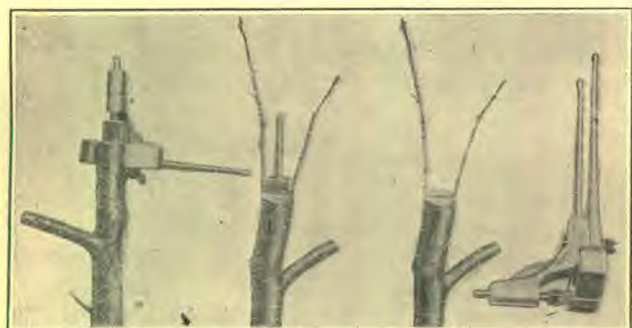
GRAFTING TOOL WHICH ELIMINATES DAMAGE TO THE BARK
