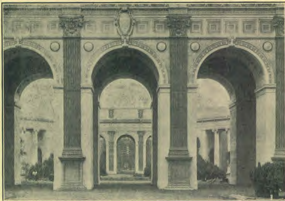
COLONNADE BETWEEN THE COURT OF THE FOUR SEASONS AND THE VENETIAN COURT
