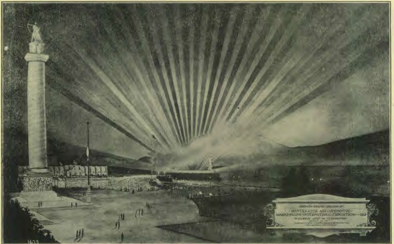
VIEW OF AN ELECTRICAL DISPLAY AT THE EXPOSITION
