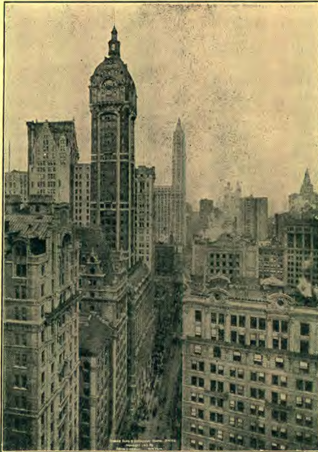
The Singer Building, as Shown in the Picture, Towers Above the Rest
