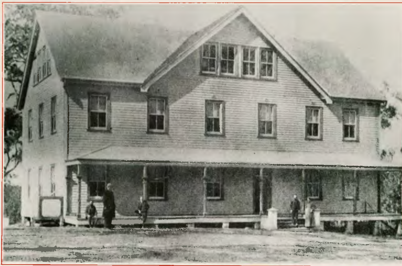
Herman Hall, the men's residence, completed in 1898. The three story building could accommodate about 80 students.
