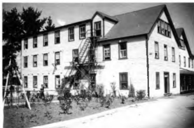
This wooden structure served as the men’s dormitory for almost seven decades, before it was replaced by Haskell Hall, named in honor of Stephen N. Haskell who led the first Adventist missionaries to Australia in 1885.
