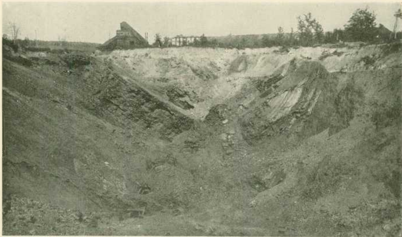
FIG. 161. A cave-in at Hollywood Colliery, Hazleton, Pennsylvania, causing what looks like a small syncline. In the Mammoth Vein. (Hardin, U. S. G. S.)
