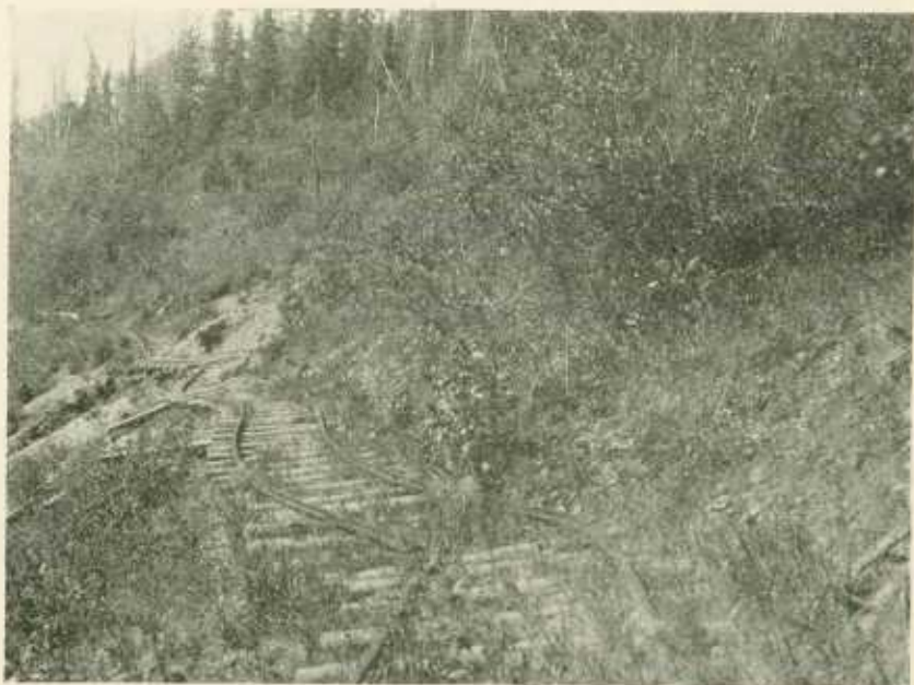
FIG. 138. Hillside creep of surface strata. The railroad is badly out of line. On a tributary of the Yukon, at Coal Creek, Alaska. (Atwood, U. S. G. S.)
