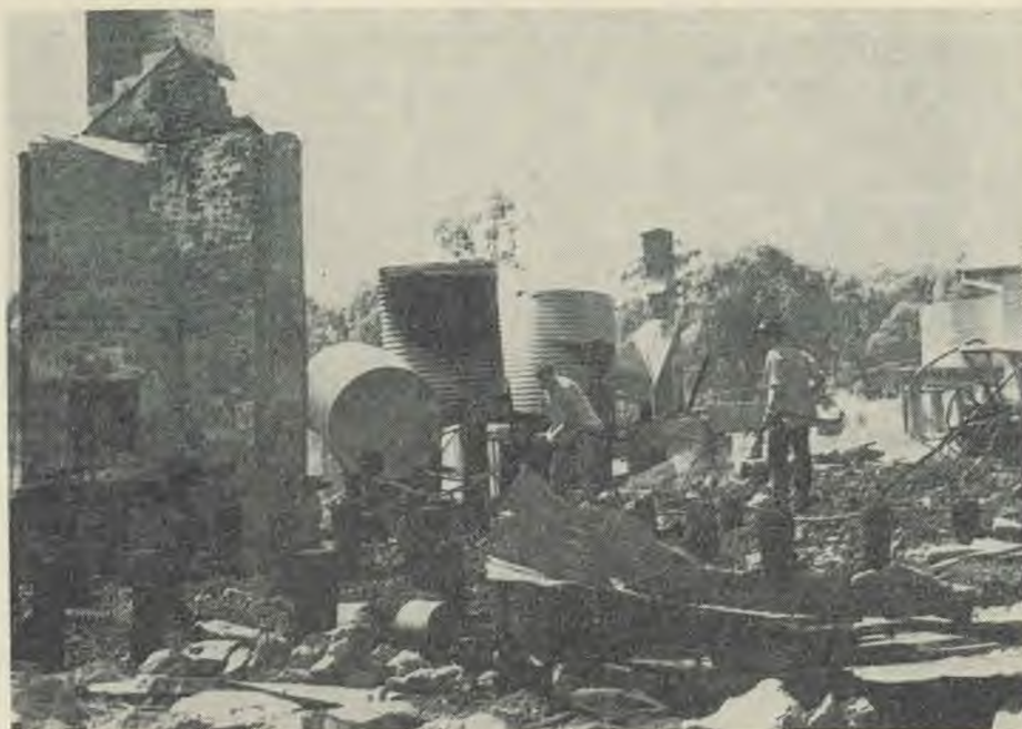
All that was left of the Melbourne family's house after the fire, which lasted only twenty minutes. (Photos, courtesy Wagga Wagga "Daily Advertiser.")
