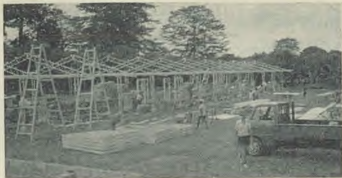
Progress after only 2½ hours' work. Such advance was possible only because of the outstanding preparation by Ray Elliott and his building team. (Photo: D. Weslake.)
