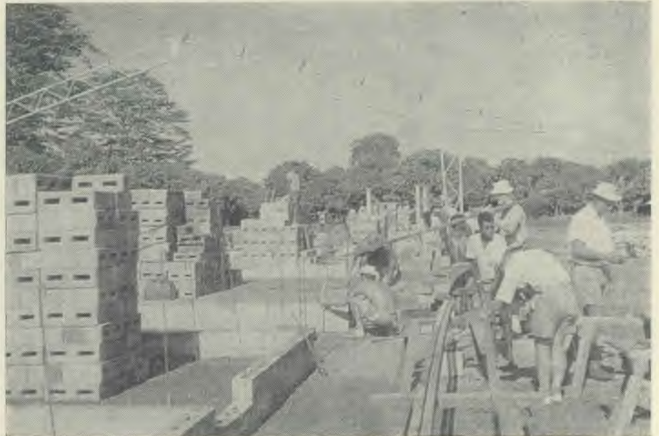
Away to a fine start. Ross Brunner (North N.S.W.) and Owen Holley (South N.Z.) lay the first of 15,000 concrete blocks. Dave Waters (North N.S.W.) and his team erect the first truss. (Photo: D. Weslake.)
