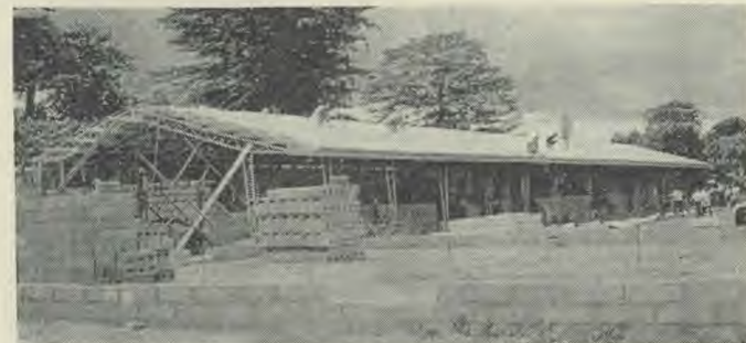
Progress at the end of the first week. Roof and walls are completed. (Photo: F. T. Maberly.)
