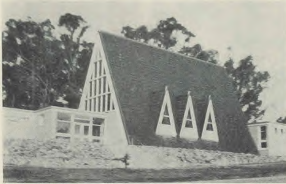
The newly constructed and now dedicated Leongatha Seventh-day Adventist church.
