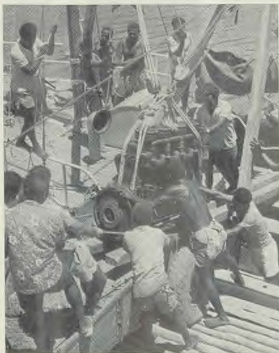
Left: Strong helpers hoist the twenty-K.V.A. Southern Cross lighting engine out from the hold of the M.V. "Laoheni." The complete unit weighed three-and-a-half tons. It was kindly made available by Mr. E. Long and his associates, of Australia. When funds are available, the hospital intends to obtain a hydro-electric turbine generator which could be harnessed to a nearby 350-foot waterfall, thus saving on fuel and maintenance costs and supplying a constant and reliable source of power.
