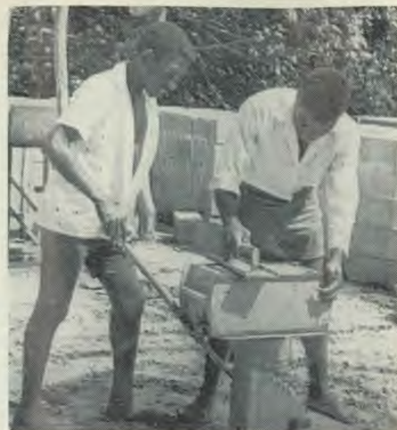
Students make concrete blocks for the new building.
