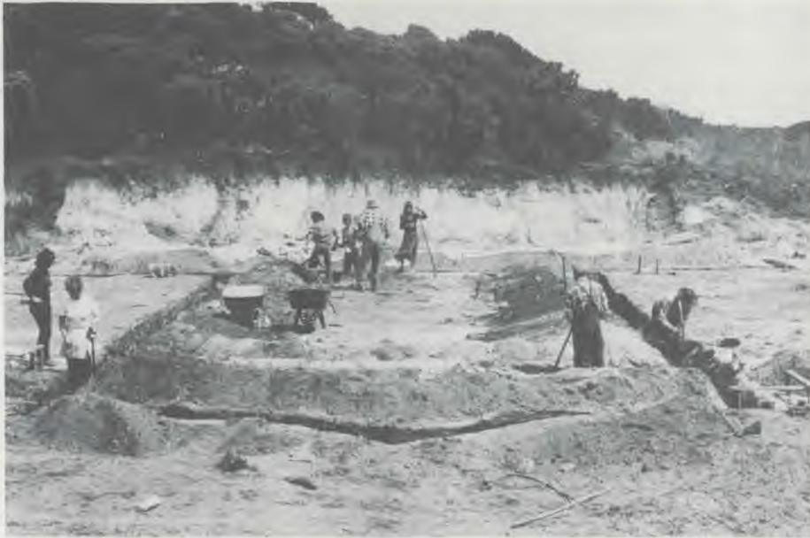
The King Island church group hard at work digging the foundations for their church. Photos: B. Whelan
