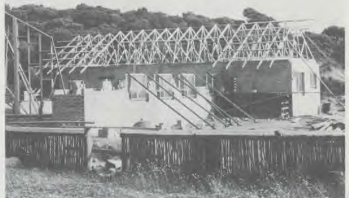
King Island's new Adventist church takes shape—this was just seven working days after commencement.
