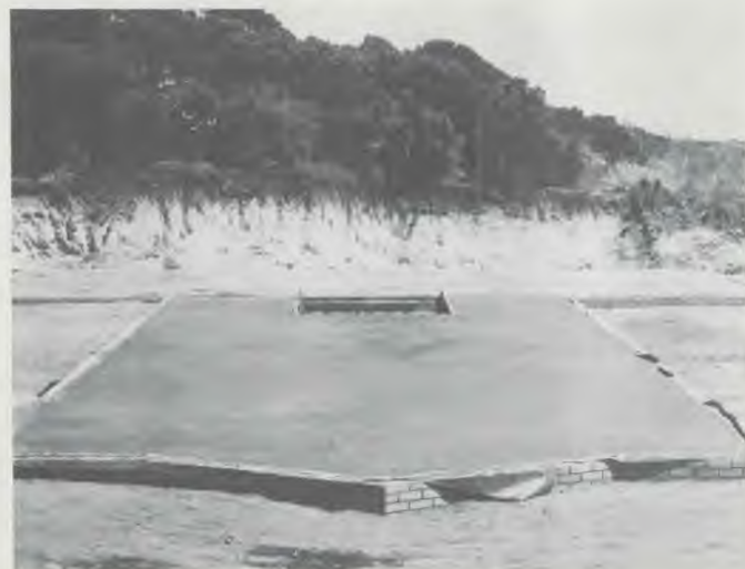
The completed concrete-slab floor—ready for the fly 'n' build team to work their sudden magic.
