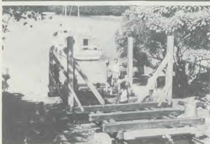
The rebuilt slipway cradle at Aore. An income-earning asset.
