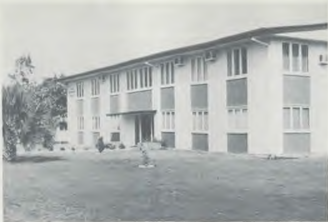
Headquarters office of the North Queensland Conference at Halliday Park, Aitkenvale, Townsville.
