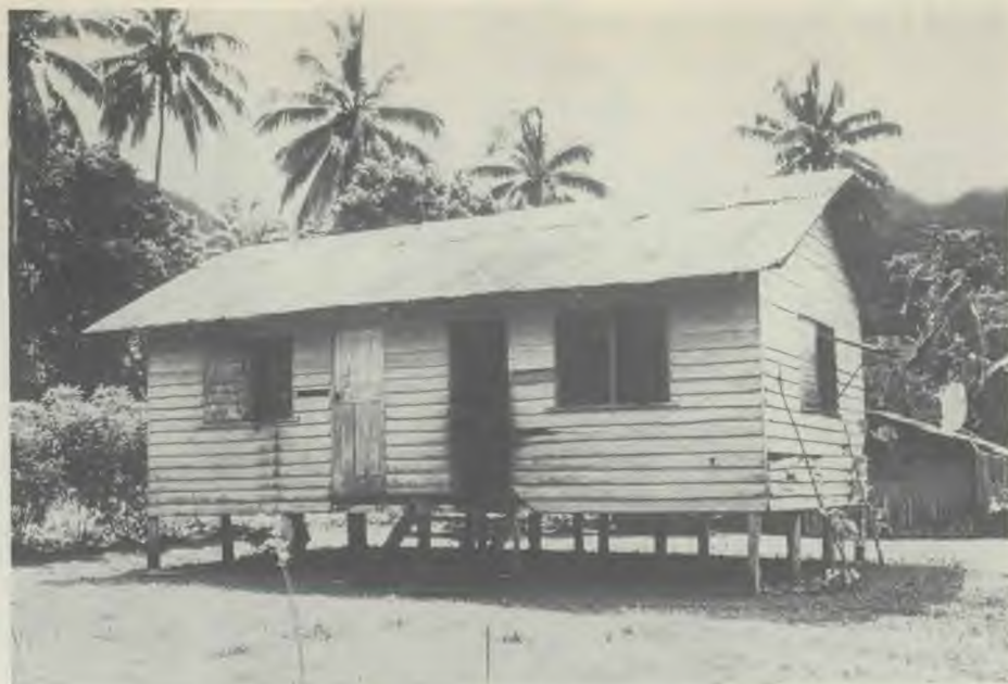
An old staff house, with a rusty, leaking roof, which badly needs replacing.
