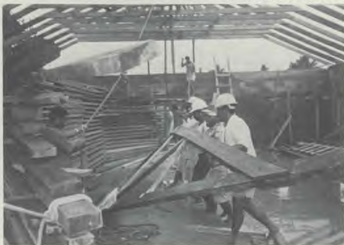
Fijian helpers handling heavy trusses for the new church at Naibita.
