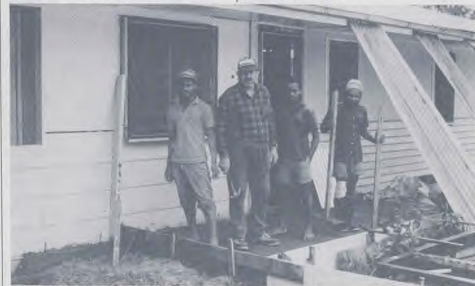
Robert Erceg, of Waitara church (Sydney), with national workers, renovate the outpatient area.
