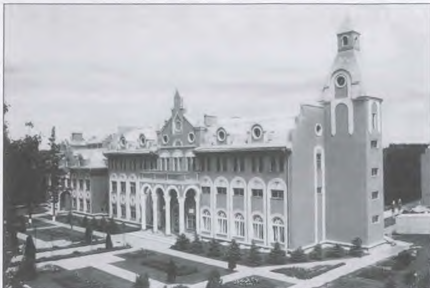
Top: Some 1800 volunteers began building the seminary in 1988. The project, the first of its kind in the Euro-Asia Division, took 20 months. Local churches decorated each of its rooms.
