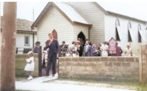
The original church building.
