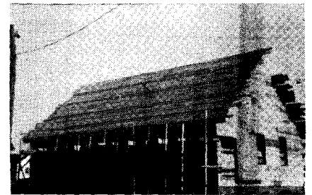
Progress of the building
