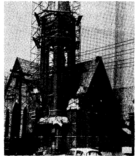
Renovating Gets Underway
