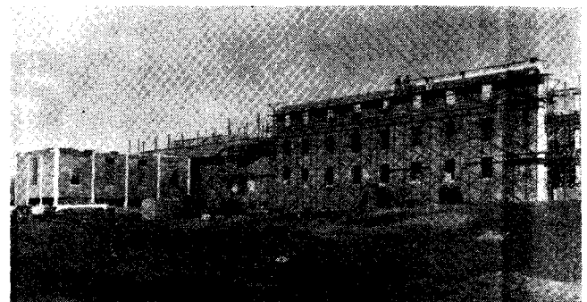
Masons lay the coping stone at roof level of boys' dormitory at Pioneer Valley Academy.
