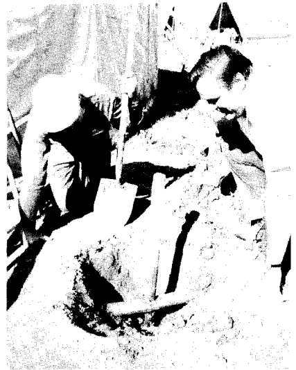
The question was, "stake or mistake?" Here Elder Ernest Stevens and Elder John Williamson locate a leak in the sewage line. A large tent stake was driven in the middle of the plastic line during camp pitch.
