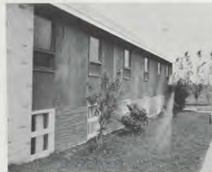
Perrysburg church after Elder Hardy Loomis installed stone work on the foundation.
