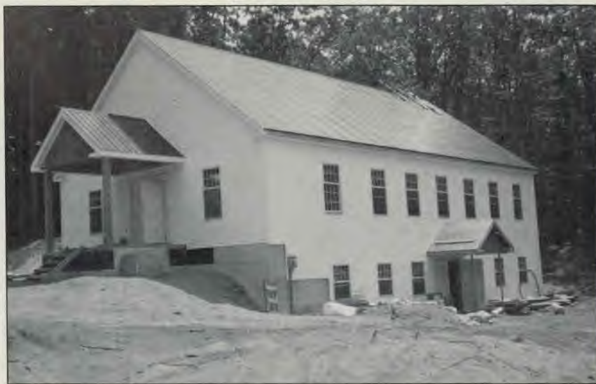
The new Snowville-Conway, New Hampshire, Church as it looked while under construction. The grounds are now beautifully completely landscaped.
