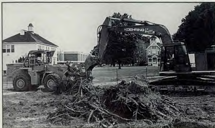
Construction of AUC's new Chan Shun Dining Commons began in mid-August. The first step was the removal of trees and leveling of the site.
