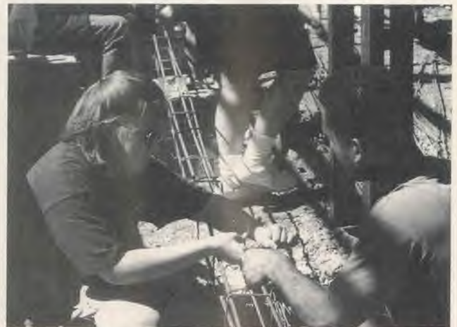
USA student Wendy Cady gets help tying rebar for bond beams from Maranatha's Dominican coordinator Manuel Crespo.
