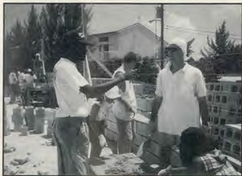
Pastor F. M. Grant (foreground) talking with construction engineer, Kendall Chaffee.
