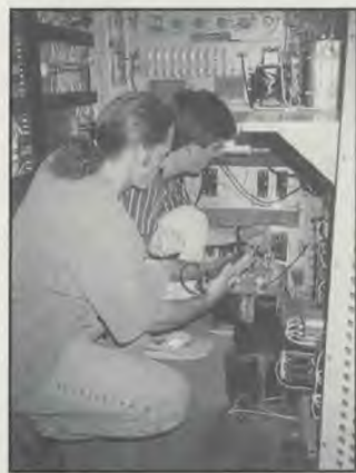
Jason Smith, engineering student volunteer, and Gary Benton, engineer, inside the new Continental 100 kilowatt transmitter.
