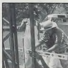
Jahni Smith, Keyonda Davis, and Teresa Roundtree running plumb lines.
