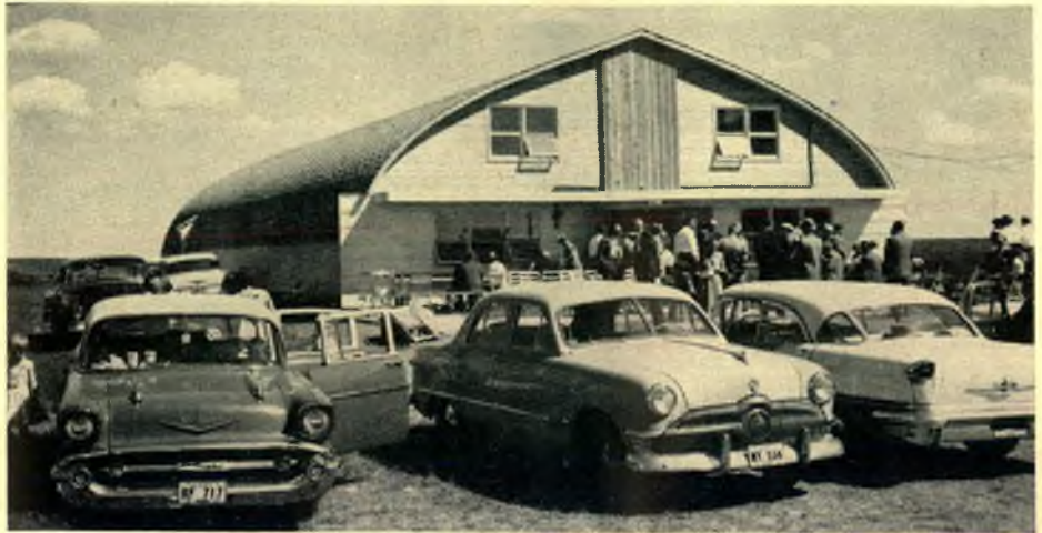
In twenty-five working days the brethren of the Rosebud church constructed this auditorium and youth centre, forty by one hundred feet, with practically no labour costs to the church. It is made to serve as an auditorium as well as a gymnasium. It is insulated and will be heated so that services can be held any time of the year. The auditorium also includes a very large, airy room for Dorcas Welfare work and storage. On the day of the Fiftieth Anniversary services one hundred and fifty cars were parked in the parking lot.
