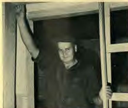
George Martni, one of the deacons, is well capable as a carpenter to perform various duties. In the picture he is seen putting in the door jams.
