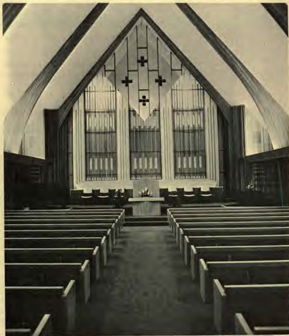
Interior view of the Westminster Church
