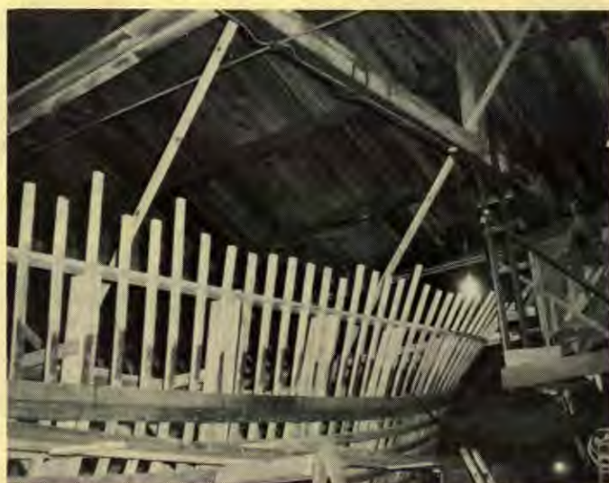
The Northern Light starts to take shape. The planking is being screwed to the stout oak ribs.
