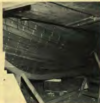
The newly installed planking on the bow of NORTHERN LIGHT.
