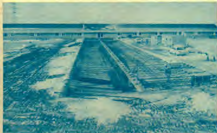
Steel being positioned in time for pouring of the floor to the 35-bed expansion.
