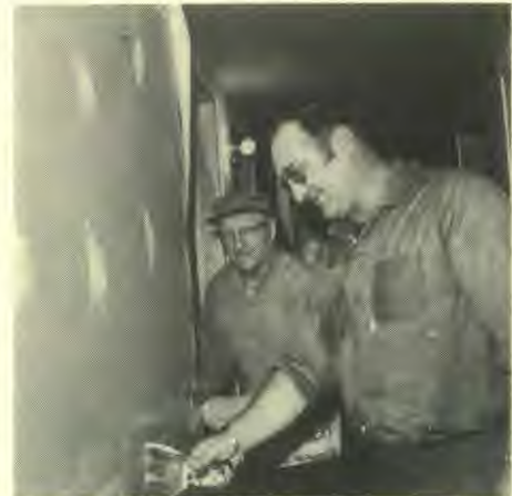
Taping and filling dry-wall in corridors — Harold Fisher, Clarence Wombold.
