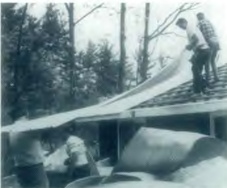
Progress on the new roof at Camp Frenda.
