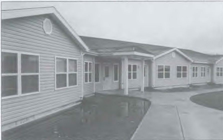
New complex awaiting spring and landscaping.
