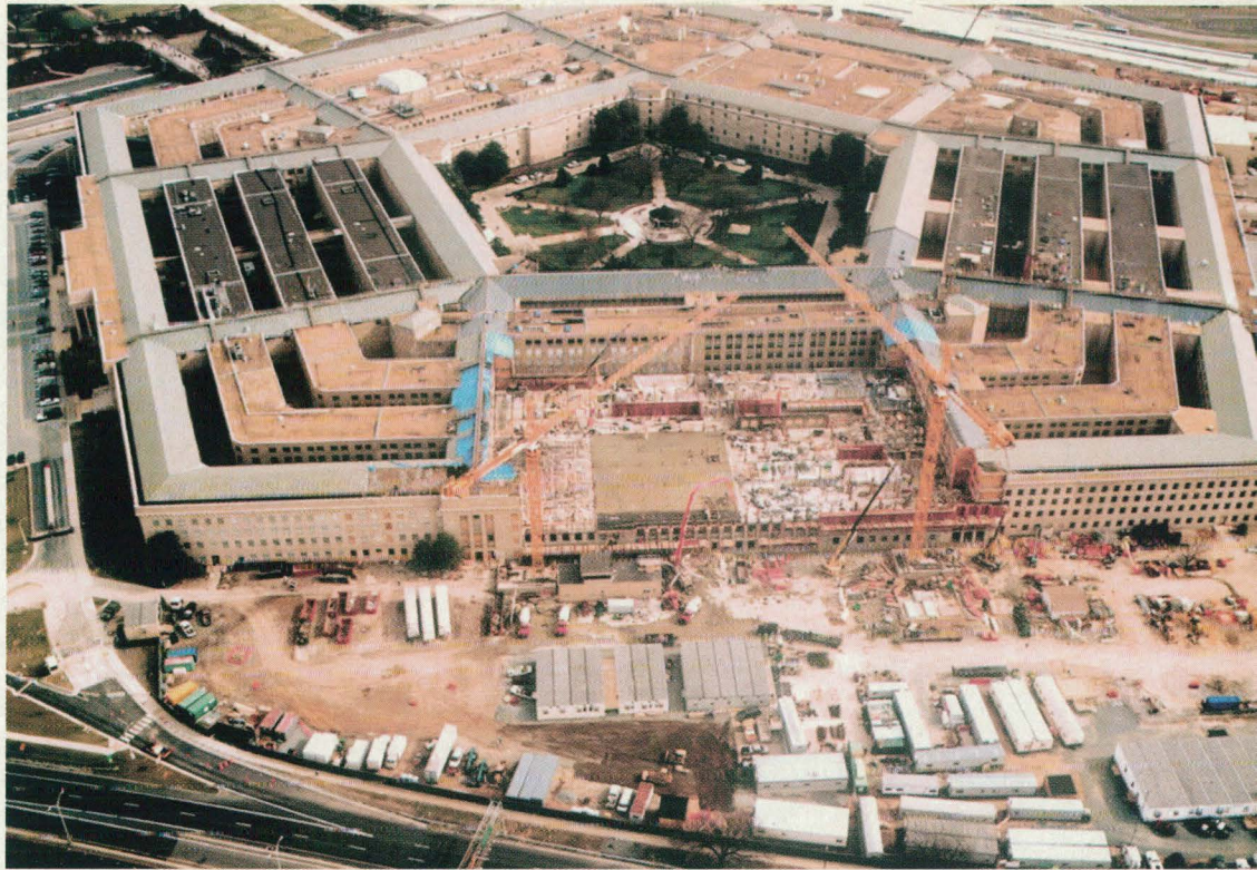
THE PENTAGON UNDER RECONSTRUCTION: Reconstruction of the Pentagon continued nearly around the clock as construction crews poured cement for floors and walls in this photo from February 6, 2002, to replace those damaged in the September 11, 2001, attack on the building.
