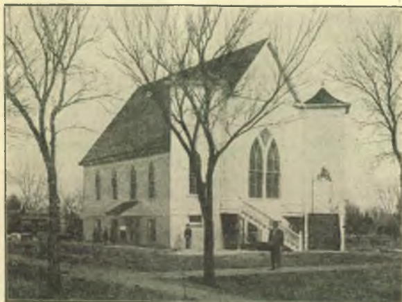
HASTINGS CHURCH—SCHOOL ROOMS IN BASEMENT.
