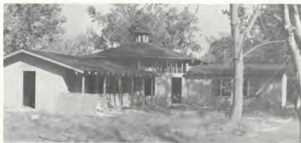
The nature center, newest building at Camp Arrowhead, nears completion.
