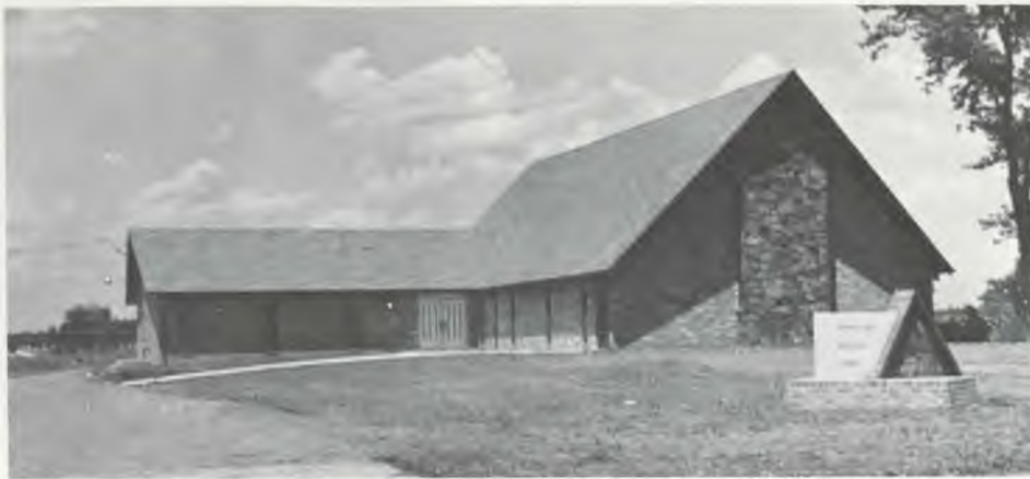
New church at Eureka, Kansas, officially opened on Sabbath, July 24, and located on busy US 54 on the east side of the city.
