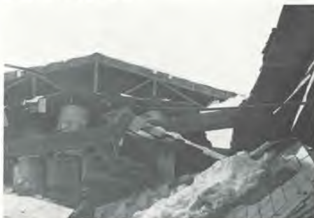
A large supply of broom corn was damaged in the roof collapse.
