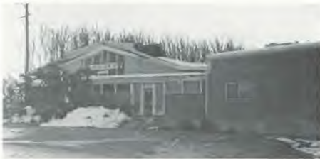
"The old broom shop" at Campion Academy will never be the same. As the result of the damage of the wet snow, it will be necessary to replace a large portion of the plant.
