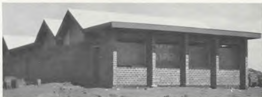
All but the brick veneer work was done in three days. A week later the brick was done.
