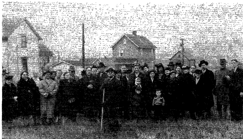
Breaking ground for Greensburg, Pennsylvania Church
