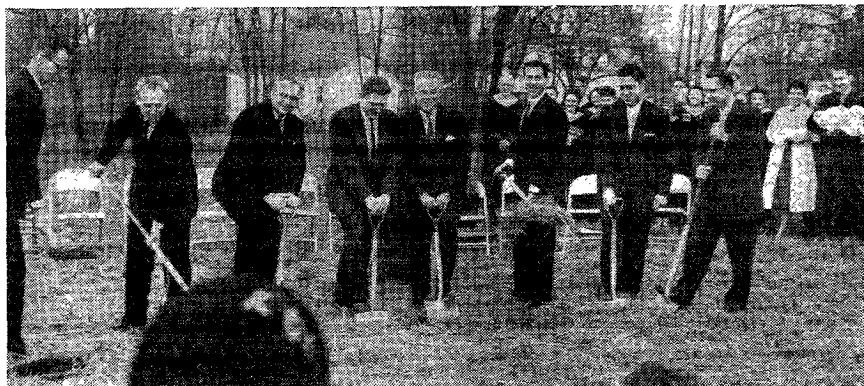
Ground-breaking for new school near Waldwick, N. J.
