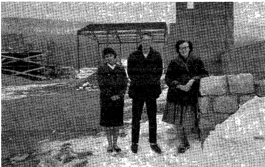
Constance Funk, Bob Yingst, and Marsha Kidder, students at Blue Mountain Academy, pose by the skeleton framework of the new Administration Building being constructed on the campus of the school. These students are typical of the 225 others who eagerly await completion of this new $400,000 facility that will house administrative offices, classrooms, the Music Department, science laboratory, Home Economics Department, and a chapel.
