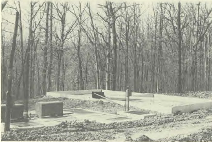
All tanks, including aerating tanks, are underground. Filter bed is on the right.
